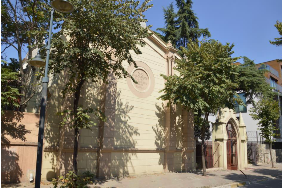
Fig. 3. The east Façade of the church
