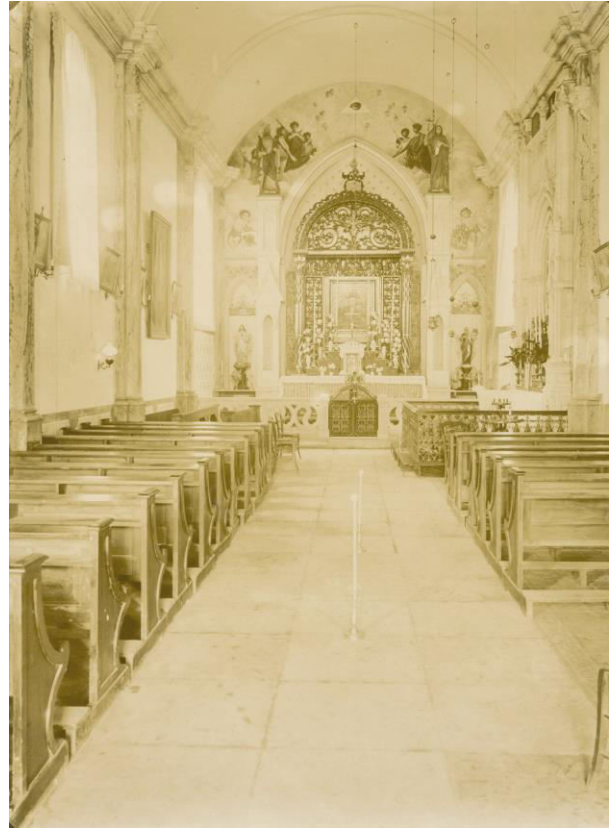
Fig. 5. The church. interior looking east (photo National Centre of Manuscripts)
