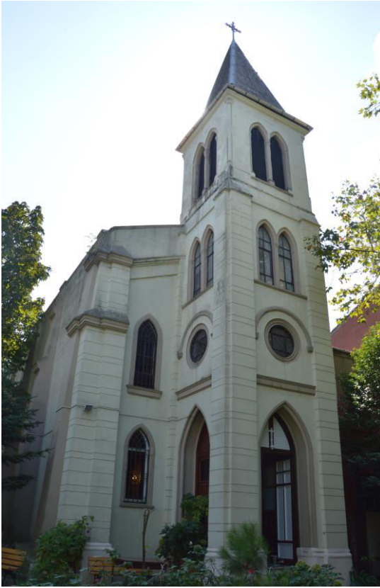
Fig. 4. The west façade of the church
