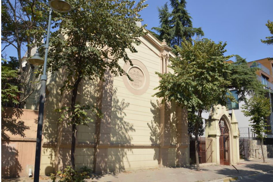
Fig. 3. The east Façade of the church
